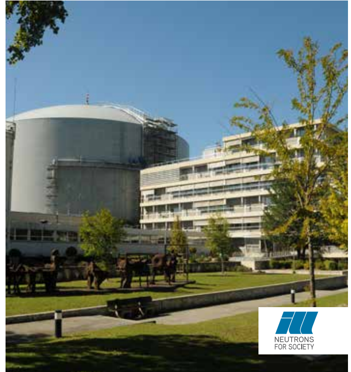
View of ILL building Credit: ILL / S.Claisse.
